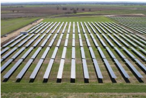
A view of the project from 125' up.
